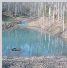
Acid Mine Drainage is frequently treated with limestone channels and settling ponds. This Natural Resources Conservation Service project treats an AMD discharge just upstream from Masontown.
